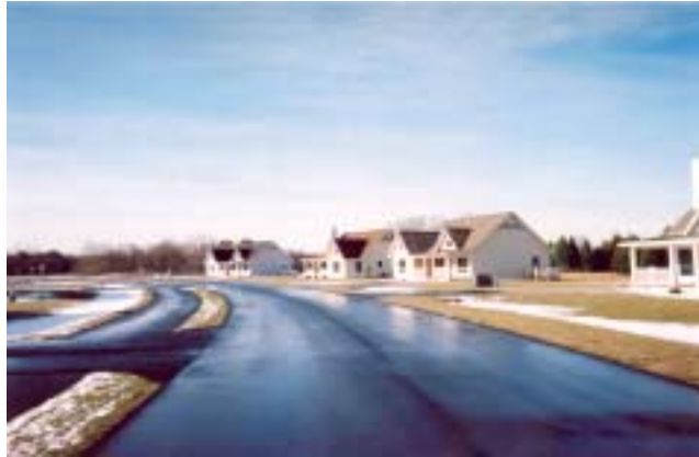
(Aki Maad zi Win completed elder units. Electrical cables, water and sewer pipes underground)
