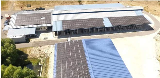
Spokane Tribe Fish Hatchery Photo Courtesy of Spokane Indian Housing Authority
