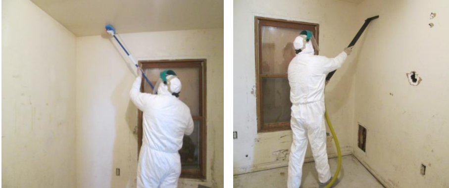
Washing a Unit with Low Contamination Levels
