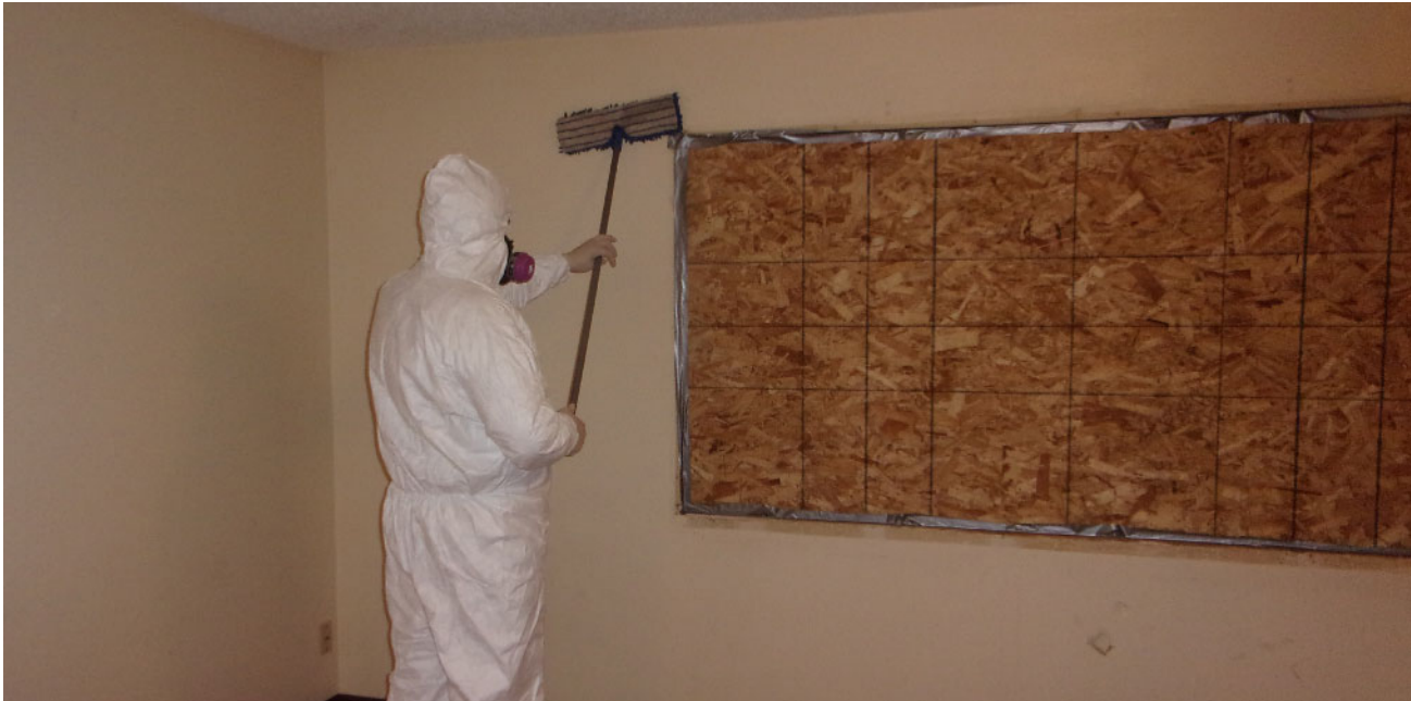
A certified remediation expert remediates a Salish & Kootenai Housing Authority unit contaminated by methamphetamine (Salish & Kootenai Housing Authority, 2021)
