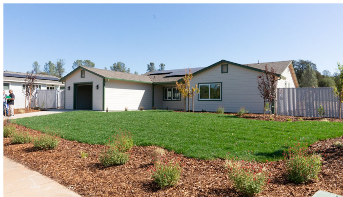
Single family homes by Mooretown Rancheria and NCIHA using HCD, & federal funds
